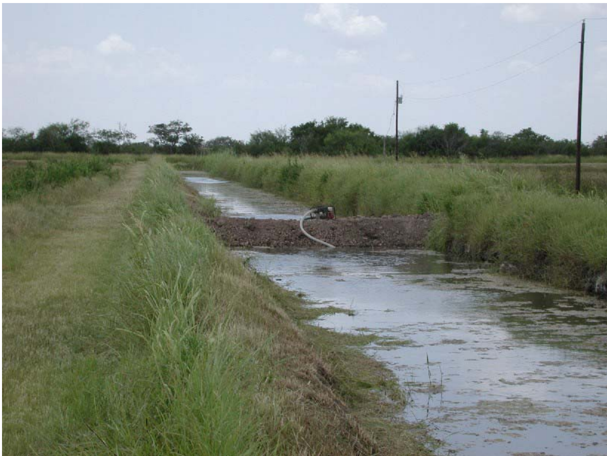
Figure 1. Earthen dam constructed on canal 55.
