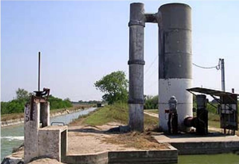
*This pump house is located southeast from the split section of the main canal and water is received through the gate structure. There are two pumps that pump the flow into the pipelines.*
