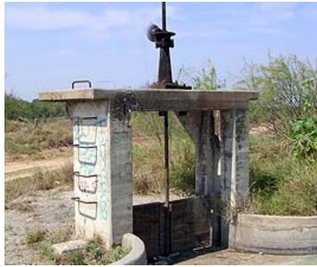
This very old head gate will be equipped with SCADA equipment and will be controlled from the Delta Lake Irrigation District Office.
